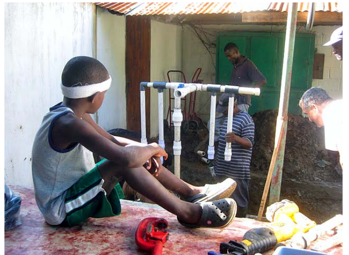
For the help that we received from HBS friends in Canada to upgrade our water system to continue to provide potable water and better serve the Limbé people.
