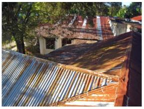
Maintenance of the facility has become an issue with most of the roofs dating back to the 60's needing replacement. Rising costs of materials and labor has forced HBS to repair only as needed. The roofs are galvanized steel on wood framework. This has become a losing battle as rotting wood and rusted through metal can only be repaired so many times. HBS needs your help to raise the monies and schedule the replacement of most of the roofs.
